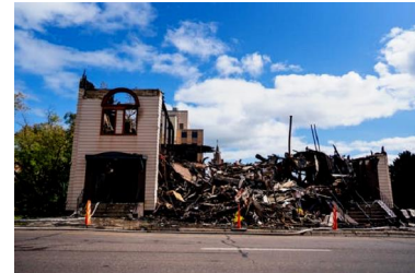
Little remained of Duluth's nearly 120-year-old Adas Israel Congregation synagogue after it was gutted by fire early Sept. 9.
